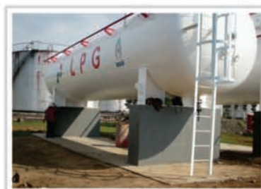
Tanki LPG 30 Ton Project SPPBE Pertamina Cepu
