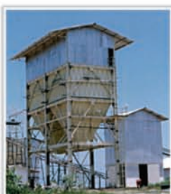
PROJECT UCI ( Lime Stone Tank )
