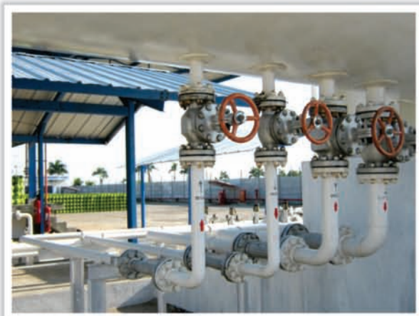
LPG Installation Piping
