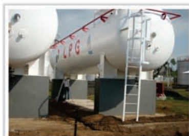
Tanki LPG 30 Ton Project SPPBE Pertamina Cepu
