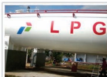
Tanki LPG 30 Ton Project SPPBE Pertamina Cepu
