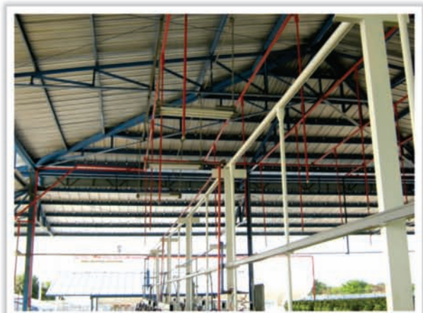
Fire Safety hydrant Installation
